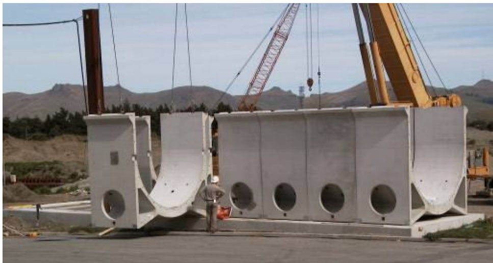
HotRot 3518 concrete modules being installed
